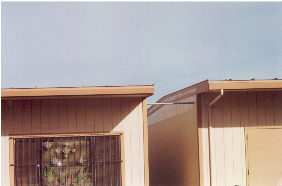
Figure 14: Conduit Running between Portable Classrooms
