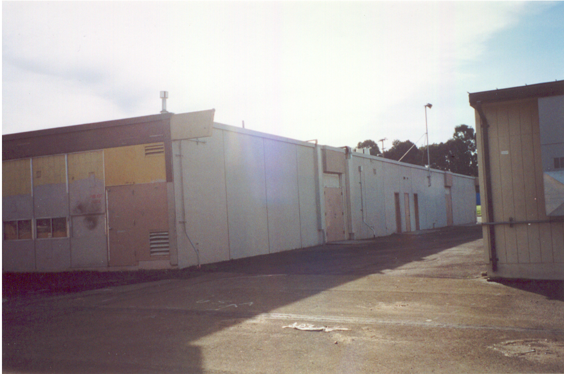
Figure 8: West Face of Main Building
