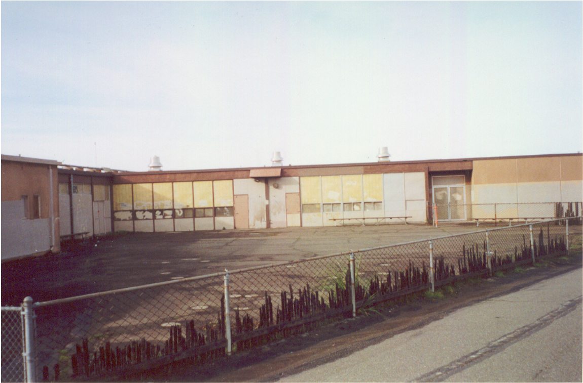
Figure 6: East Face of Main Building
