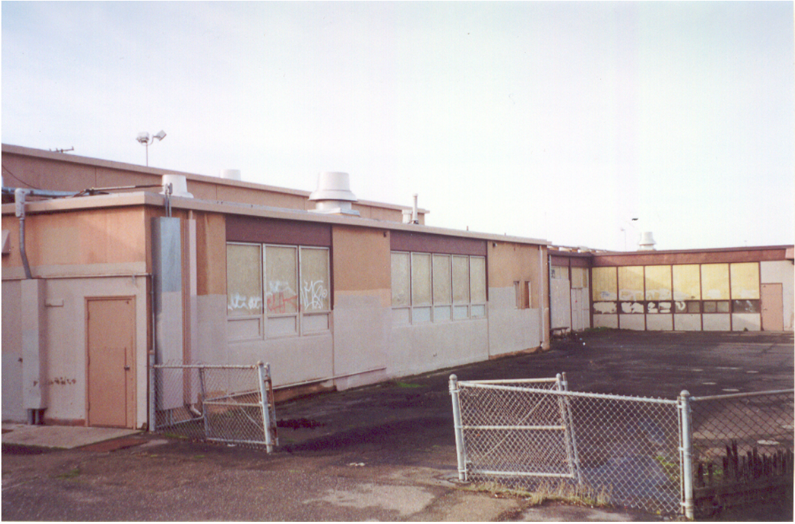
Figure 5: North Face of Multi-Purpose Building at Kitchen Area
