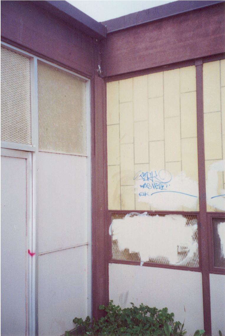
Figure 16: Seismic Joint at Corridor near Main Building
