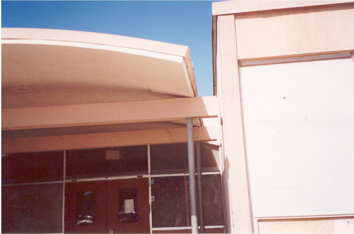
Figure 15: Entrance Canopy at Main Building
