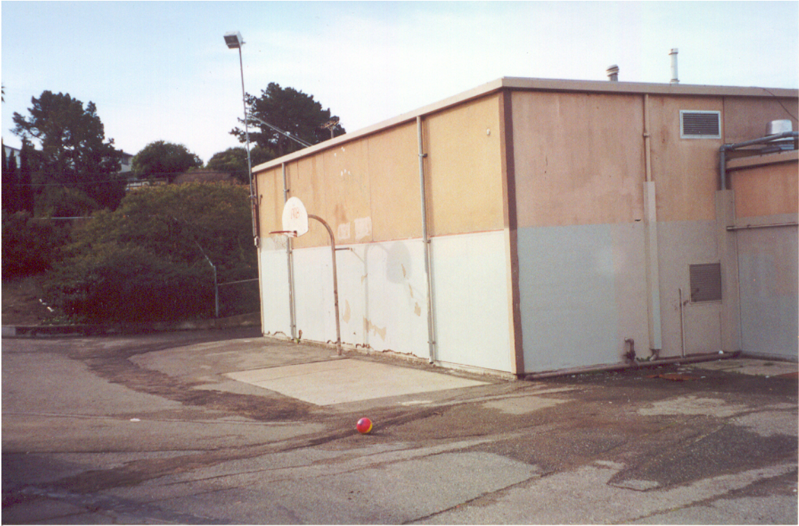
Figure 4: East Face of Multi-Purpose Building
