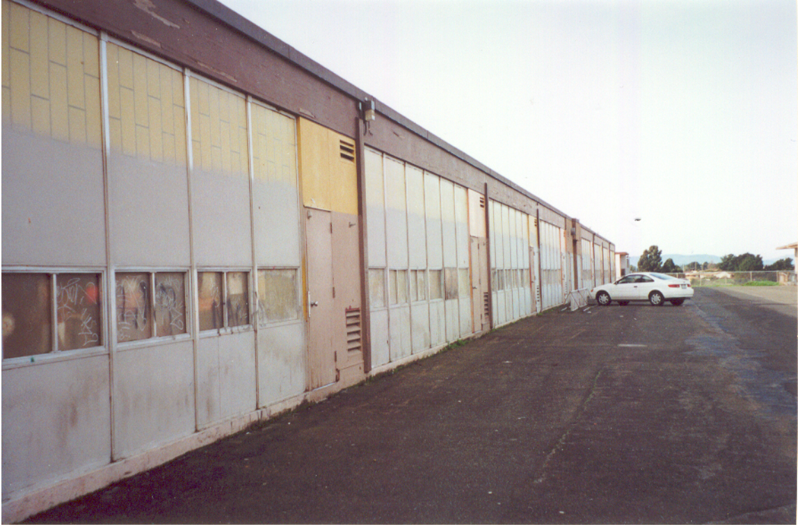
Figure 7: North Longitudinal Wall of Main Building
